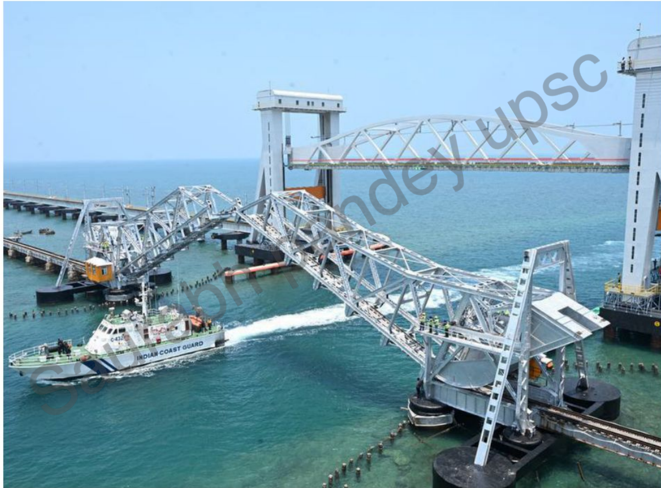
A Coast Guard vessel passes through Pamban channel as Railway authorities lifted the vertical span of the New Pamban Rail Bridge during a
