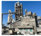
This is General's Alexandria Portland Cement Company factory in the Mediterranean city of Alexandria, Egypt. Reuters
