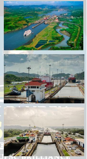
The Canal's locks at each end lift ships up to Gatun Lake, an artificial freshwater lake 26 meter above the sea level created by damming the Chagres River and Lake Alajuela to reduce the amount of excavation work required for the canal, and then lower the ships at the other end.
